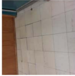
CES replace floor in multipurpose room
