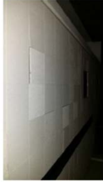
CHS, SMS Replace ceiling tile and ACM abatement (SMS)
