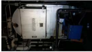
CPS Install new boiler - CT
