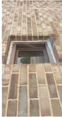
CHS Replace Library Windows CT
